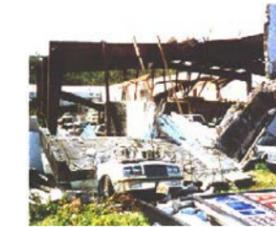
Poorly reinforced hollow-block walls can topple
